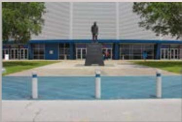
The Century precast concrete security bollards can be manufactured with custom designs and colors to aesthetically blend in with the architectural surroundings while effectively preventing vehicles from running through building entrances and on pedestrian sidewalks.
