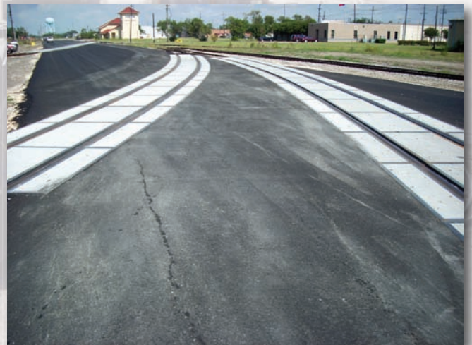
Concrete Railroad Grade Crossings in Spiral Curve
